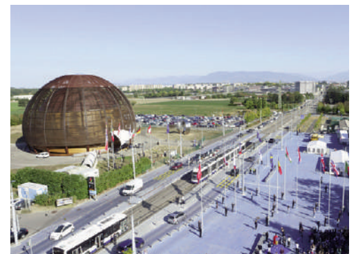
Fig. 8 | Aerial view of the territory occupied by the CERN plants, with underground tunnel tracks, June 1986 (credit: J.-L. Caron, CERN Photos Archive).
