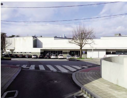
Fig. 1 | 'Escola Secundária Sá de Miranda' in Braga by Bernardo Távora: new building to enhance and accentuate the importance of the pre existence in the urban fabric (credit: A. Santos, 2012).
