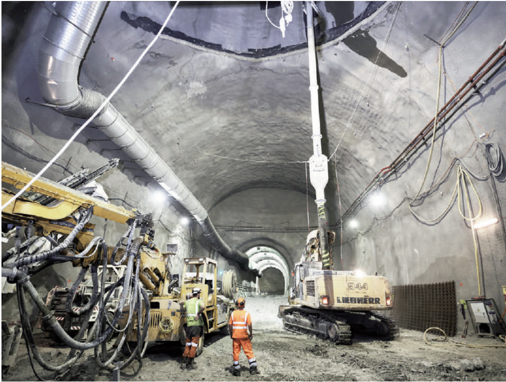
Fig. 7 | Tunnel work for the future High Luminosity Large Hadron Collider (HL-LHC), 16 August 2019 (credit: M. Brice, CERN Photos Archive).
