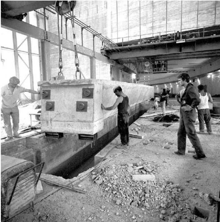
Figg. 4, 5 | The Intersecting Storage Rings (ISR): construction of the main base; laying of a magnet module (credits: CERN Photos Archive, 1969).
