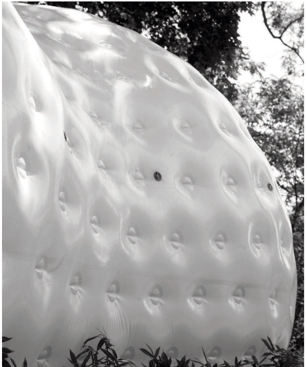
Fig. 13 - Modern Tea House (Kengo Kuma, 2007), building with air (credit: Archivio Form TL).
