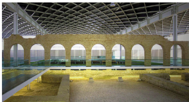
Figg. 7, 8 - The Roman Villa La Olmeda in Palencia, Spain: the wide metallic structure of four vaulted roof modules designed by Parades Pedrosa Arquitectos in 2009 (credit: Roland Halbe).
