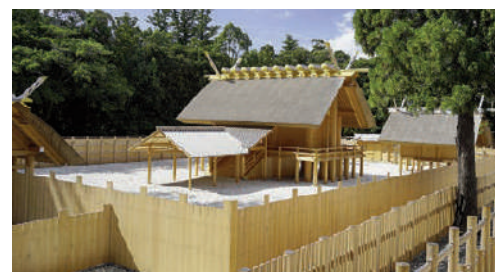
Figg. 5, 6 - The Great Shinto Shrine of Ise rebuilt on the occasion of its 62nd anniversary in 2013, according to a well-established practice that since the seventh century has been repeated every twenty years (credit: Ise-Schrein).
