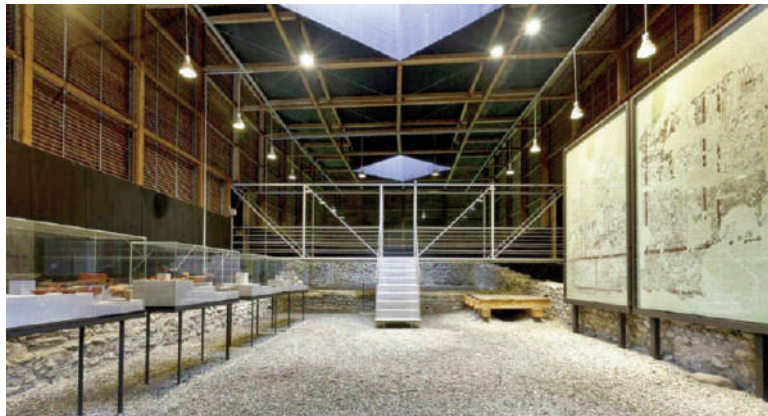
Figg. 13, 14 - The Roman archeological excavations in the area of Welschdörfli in Chur, Switzerland. The envelope horizontal texture, designed by Peter Zumthor in 1985, is composed of horizontal wood timbers that shade the sun while allowing air in and suggest a temporary form in contrast with the permanence of the stone ruin inside (credits: clemsoningenoa; Felipe Camus).
