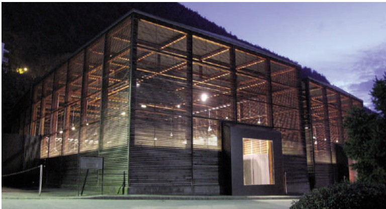
Figg. 13, 14 - The Roman archeological excavations in the area of Welschdörfli in Chur, Switzerland. The envelope horizontal texture, designed by Peter Zumthor in 1985, is composed of horizontal wood timbers that shade the sun while allowing air in and suggest a temporary form in contrast with the permanence of the stone ruin inside (credits: clemsoningenoa; Felipe Camus).
