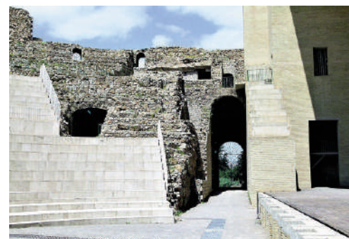
Fig. 22-24 - The ruins of the Roman Theater of Sagunto, Spain, and its reconstruction designed by Giorgio Grassi (1985-1993).
