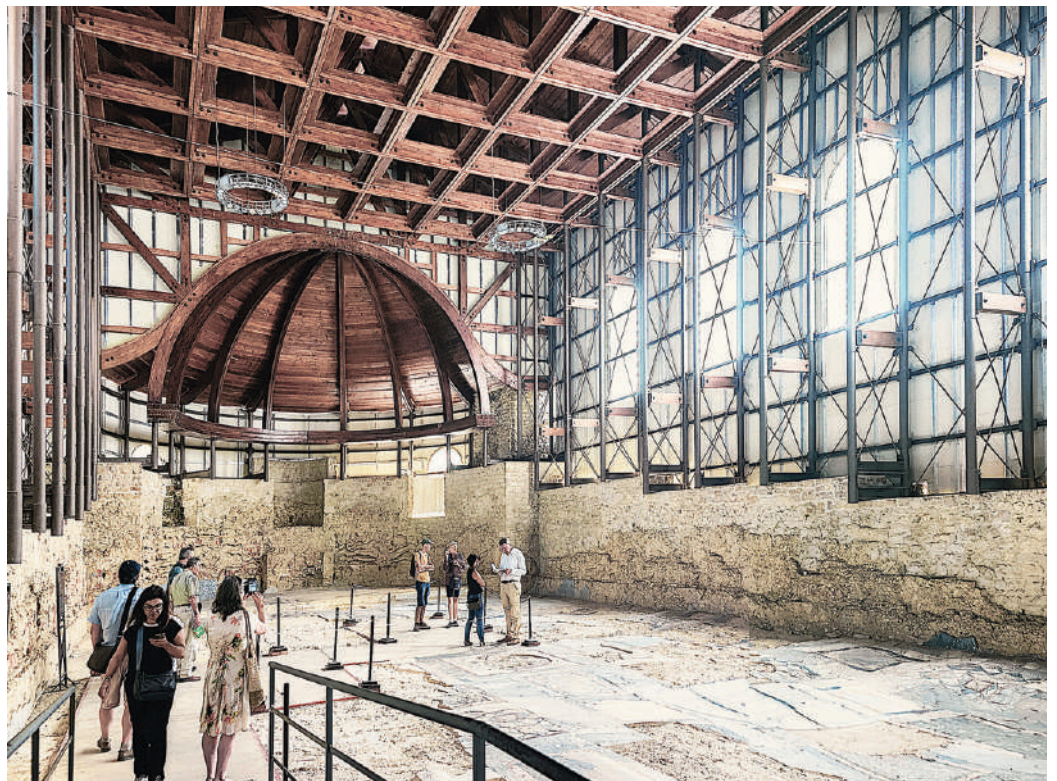
Fig. 27-29 - The Villa Romana del Casale in Piazza Armerina, Sicily, Italy: the reconfiguration projects designed by Franco Minissi (1956-1967) and the Istituto Centrale del Restauro one (2004-2012); the recent one resolves the problems of conservation performance, lighting and visitor circulation, and improves the visitor experience (credit: Roman Babakin/Alamy Stock).
