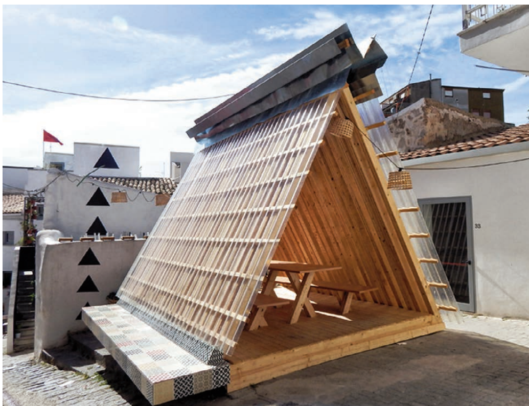
Fig. 19 - Equilatera, a pavilion in scraps of X-LAM for the courtyards of Farm Cultural Park (credit: Politecnico di Milano).
