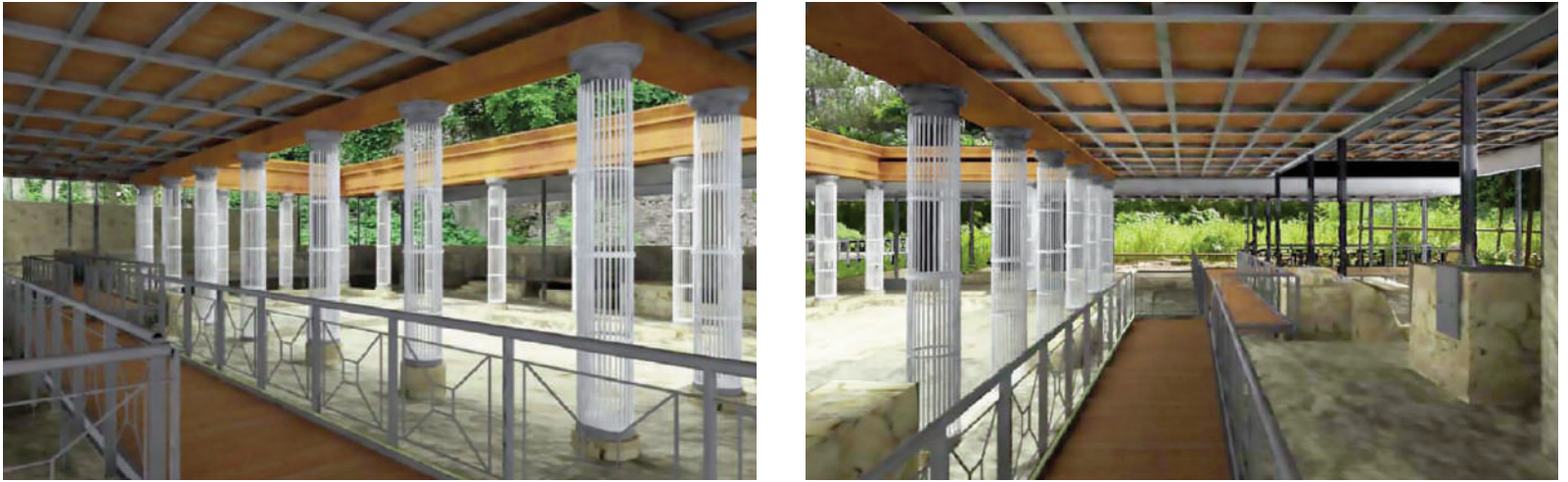
Fig. 30, 31 - The Villa Romana San Pancrazio in Taormina, Sicily, Italy: the project of the protection shelter designed by Alberto and Cesare Sposito (2005), with the evocative reconfiguration of the peristyle and the walkway systems for the fruition of the mosaics (credit: Authors).
