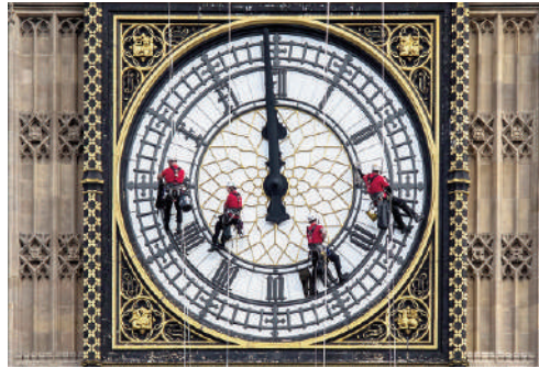
Fig. 7 - Big Ben Clock in London, under continuous maintenance (credit: UK Parliament/Stephen Pike).
