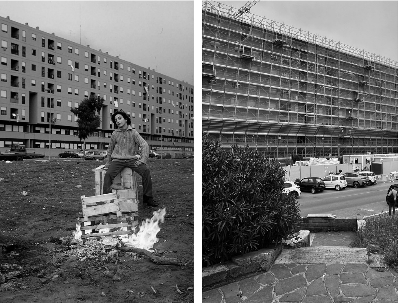
Fig. 13 | Image of Tor Bella Monaca (Rome) shortly after completion and image of the current construction site (credits: T. Garbasso and E. Cangelli).
