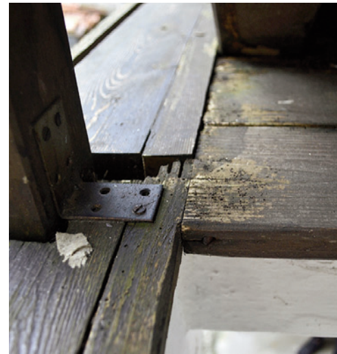
Figg. 5-7 | Details: the exfoliation phenomenon of the protective varnish on the wooden elements of the Daltz; the photochemical oxidation phenomenon on wooden balconies; the discovery of boreholes indicating the presence of insects (credits: I. Zamboni, 2023).
