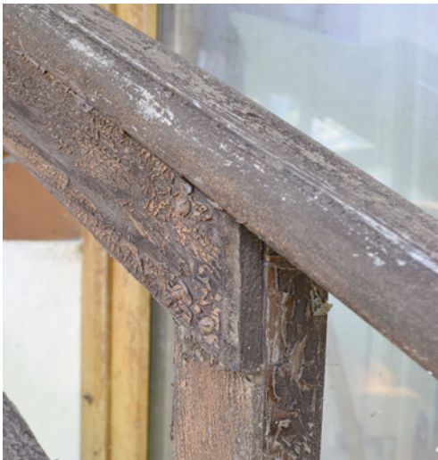
Figg. 5-7 | Details: the exfoliation phenomenon of the protective varnish on the wooden elements of the Daltz; the photochemical oxidation phenomenon on wooden balconies; the discovery of boreholes indicating the presence of insects (credits: I. Zamboni, 2023).
