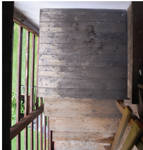
Figg. 5-7 | Details: the exfoliation phenomenon of the protective varnish on the wooden elements of the Daltz; the photochemical oxidation phenomenon on wooden balconies; the discovery of boreholes indicating the presence of insects (credits: I. Zamboni, 2023).
