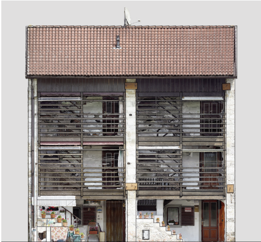
Fig. 11 | View of the existing state of the building based on the ortho-mosaic photograph obtained by photogrammetry (credit: V. Riavis, 2024).
