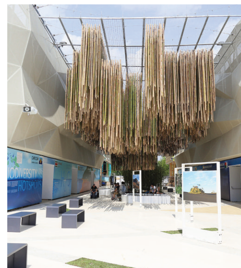
Figg. 5-8 - Islands, Sea and Food Cluster pavilion at ExpoMilano2015; engineered by Atelier2 and LAPS Architecture, between Milan and Paris; built by RUBNER ObjectBau.
