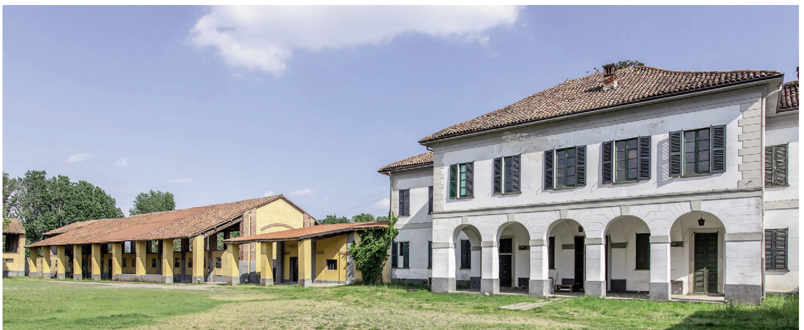
Figg. 5, 6 | Cascina Ri-Nascita: state of affairs: large and small stable; status quo, the manor house, the former clubhouse, and the large stable (credits: T. Della Frana, 2023).
